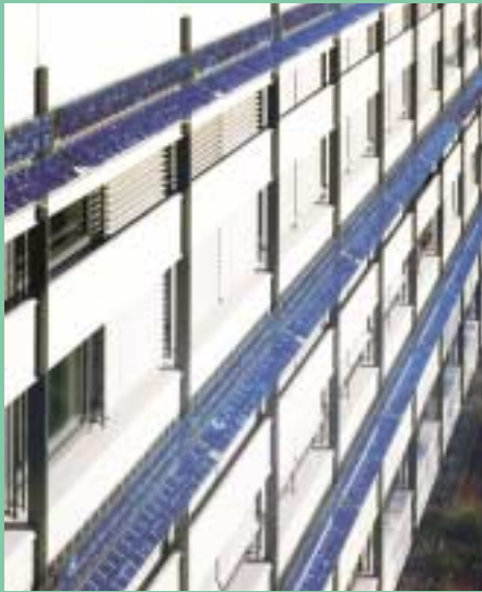
Examples of PV systems used as a shading device for an office building (above) integrated into a vertical surface at Fraunhofer ISE Freiburg (below) and installed into an atrium, at the University of Florence, Italy (bottom)
