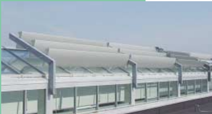
Shading devices at Aabenraa Hospital.
