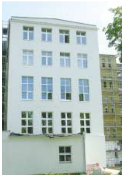
100 mm exterior insulation used for Torun Hospital.
