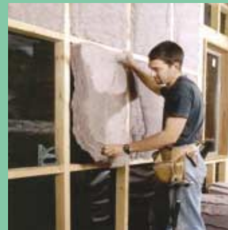
Installation of wall insulation
