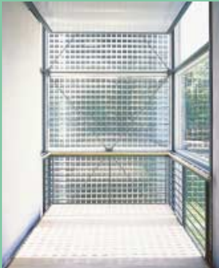
Examples of PV systems used as a shading device for an office building (above) integrated into a vertical surface at Fraunhofer ISE Freiburg (below) and installed into an atrium, at the University of Florence, Italy (bottom)
