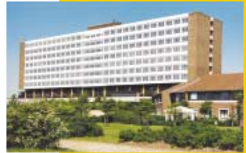
1+2 Window Outside 1-layer glazing Void with integrated sunscreen Inside 2-layer energy glazing
